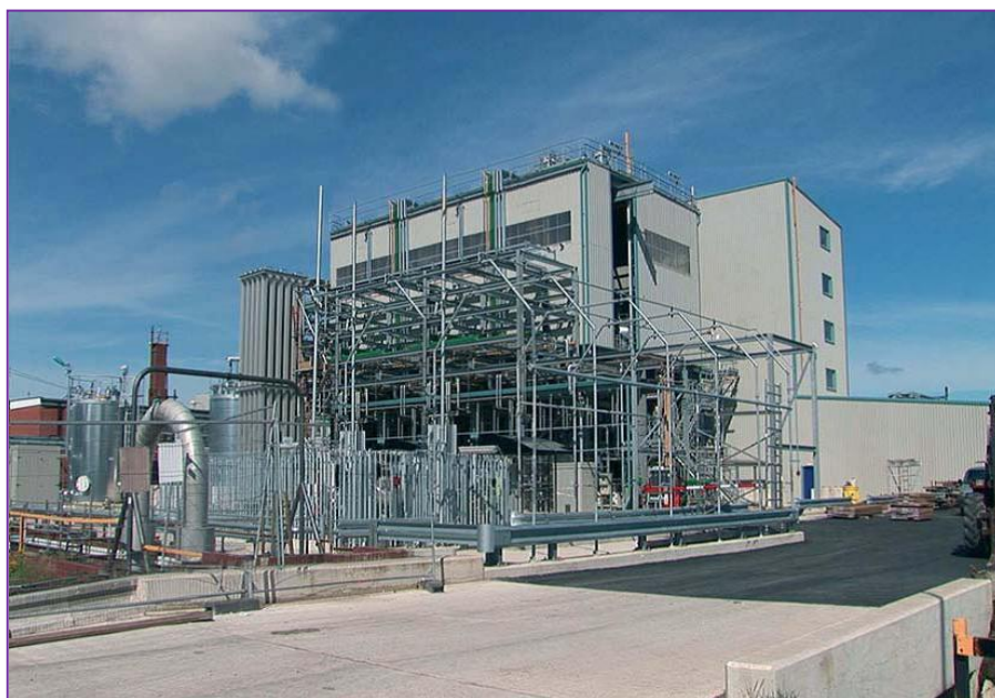
Hillhouse Technology Enterprise Zone, Thornton
